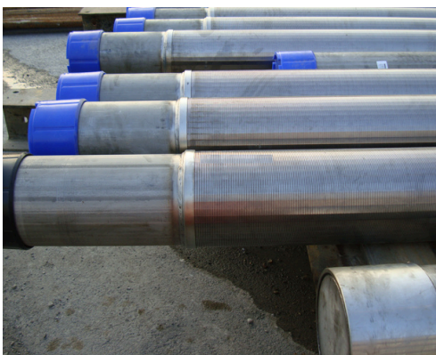
Filter screens ready for installation in the well
